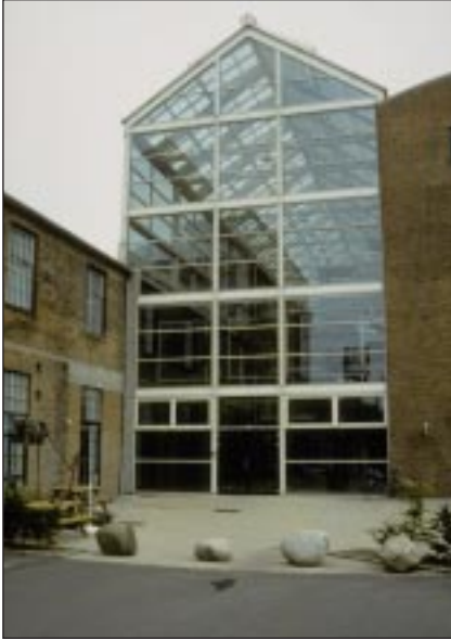
Figure C.3 The atrium west end wall seen from outside.
