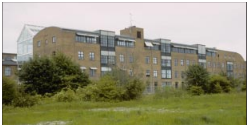
Figure C.4 The A building seen from the South.
