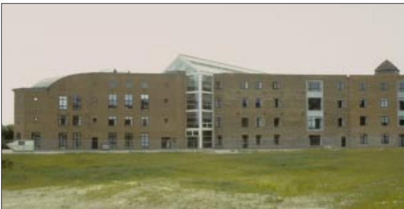
Figure C.1. The K+A building and the atrium seen from the East.
