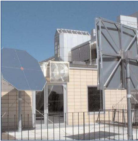
Heliostat-based lighting system
